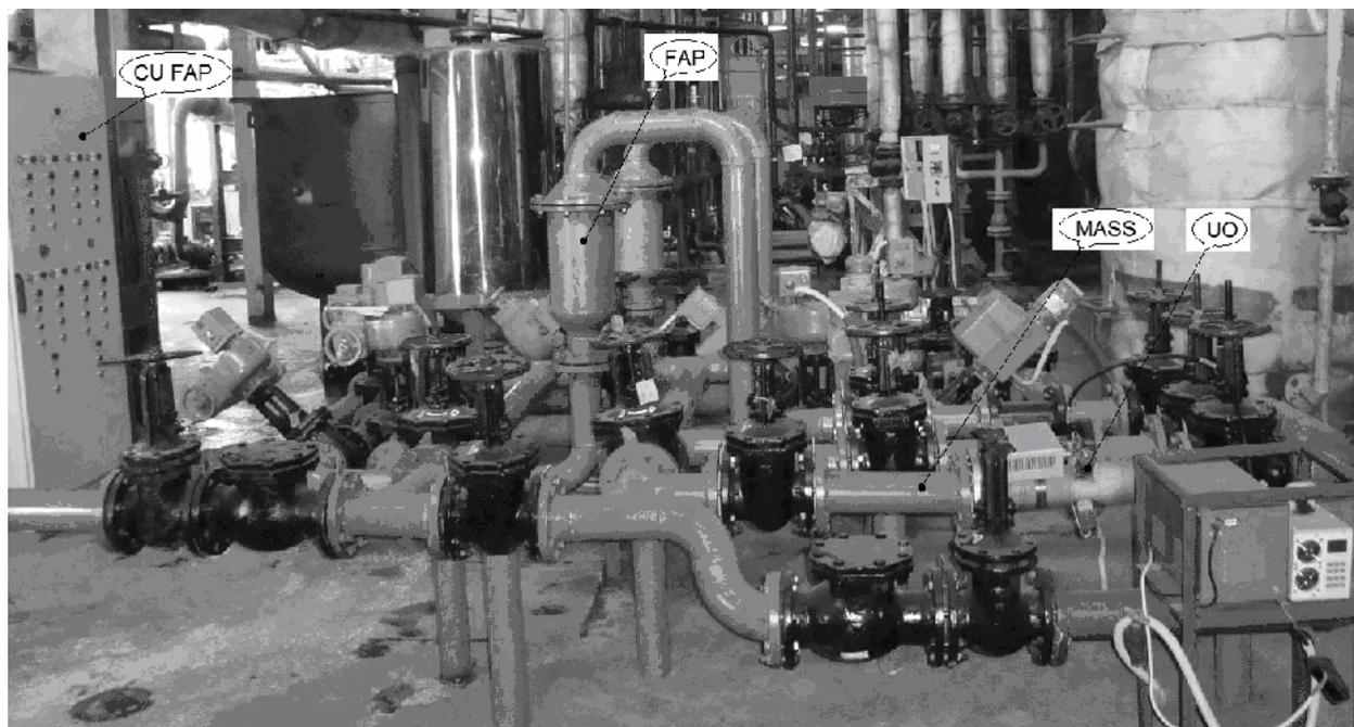
Fig. 1. The ultrasonic magnetic adsorptive system of water purification
